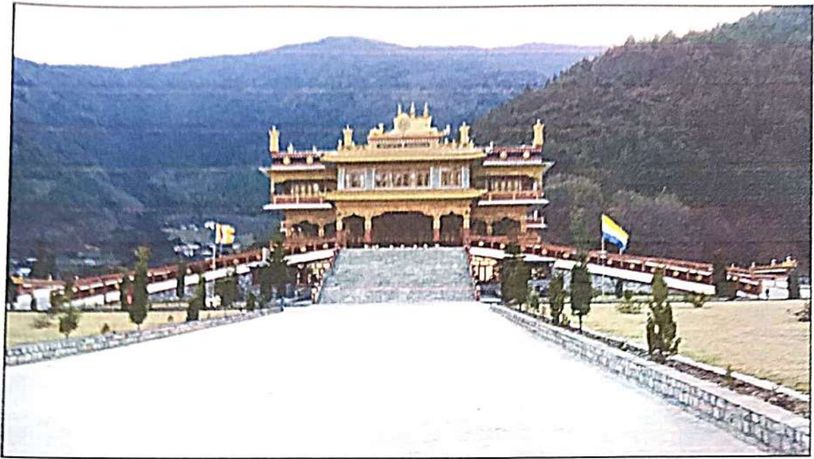
Photo No. 4.1: Thupsung Dhargyeling Monastery, Dirang.
